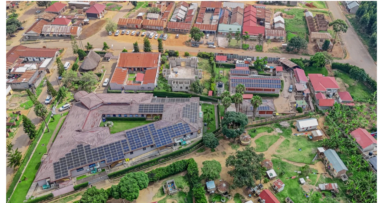
Solar system at RHSP Headquarters in Kalisizo.
